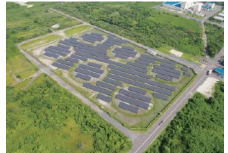
Kudamatsu Mega Solar Power Plant
