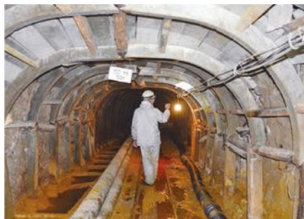
Gallery inspection at Hanawa Mine
