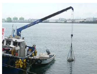
Installation of blocks for the epiphytic growth of algae
