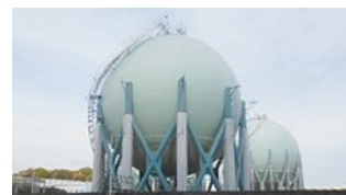
Brace retrofitting on a spherical tank
